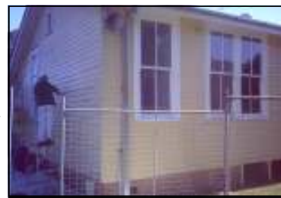
P1 & P2—1st to get a coat of paint
